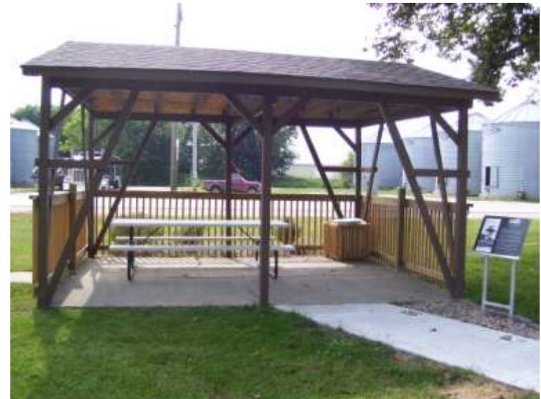
Refurbished shelter house at Triangle Park. Hwy 175 and Main
